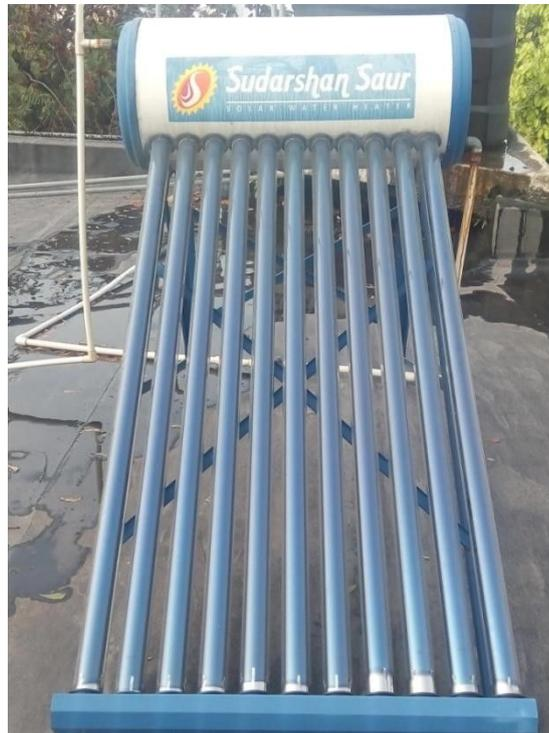
**Figure 2.1** Evacuated Tube Solar Water Heater
